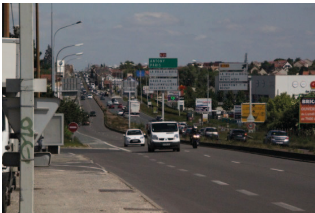
The RN20 and the project to create a dedicated on-site public transportation network.
