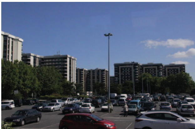
Grigny II and the deteriorating condominiums
