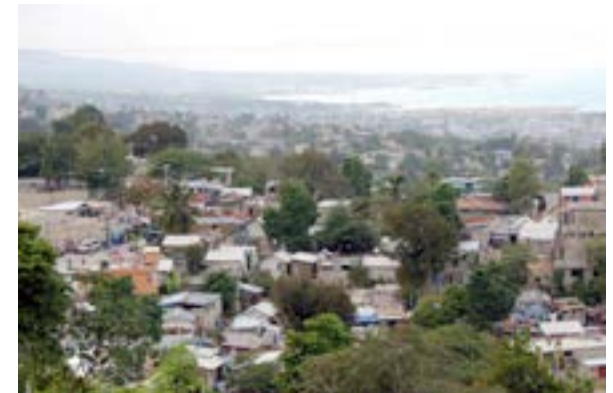
Port-au-Prince, constructions informelles
