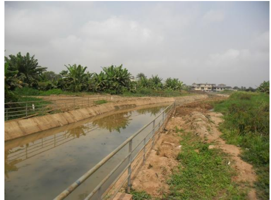
The branch of the G collector crosses the Donoukin and drain the city's rain and waste water.
