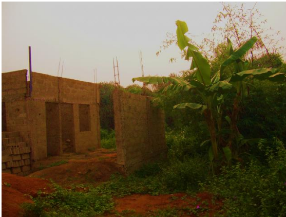
A house under construction in the depression
