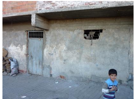
Ground floor areas are used as sheds. Will they be used as garages?
