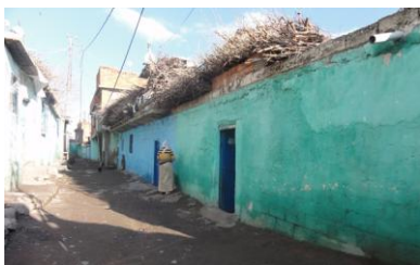
Bundle of firewood stocked on the roof for the heating system.
