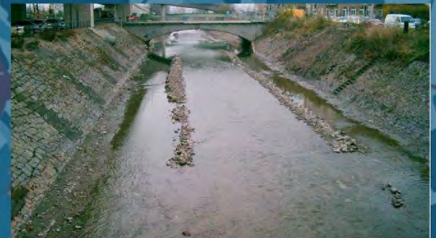
Enlargement of riverbed cross section in response to flood hazards of Weisseritz river (City of Dresden – Environmental Office 2023)
