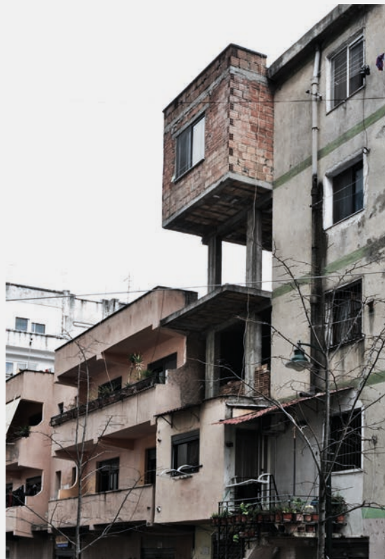
Informal addition to existing building
