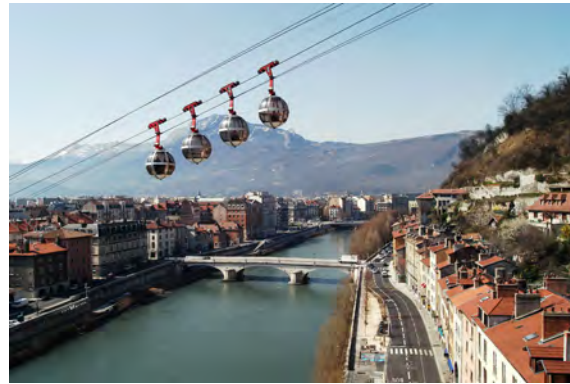
Téléphérique de la Bastille, Grenoble A cable car with translucent “bubbles” and over 14 million visitors
