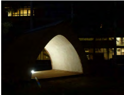
Wood+earth+straw vault, Neuville Campus Participative work with students of the IUT Génie Civil
