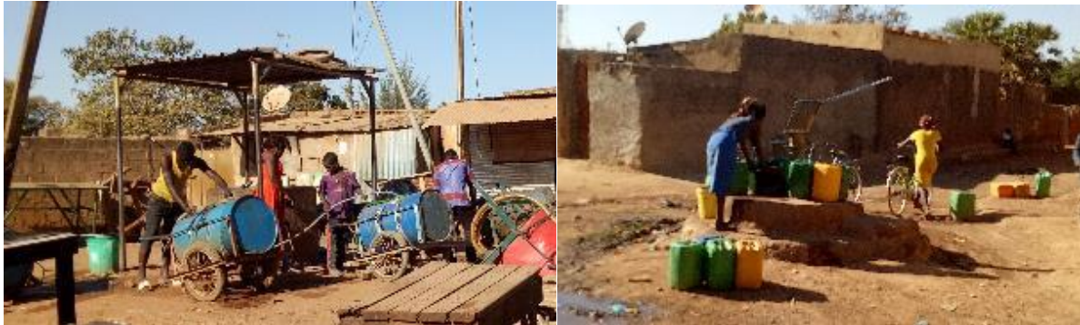
Figure 16: A standpipe (left) and a borehole (right) in the non-loti area of Somgandé
