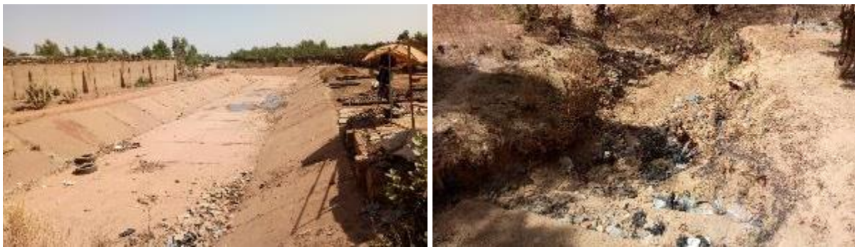
Figure 24. Portion of the drainage outlet developed in the loti area south of the RN3 (left) and a portion of the undeveloped outlet in the non-loti section of Kossodo
