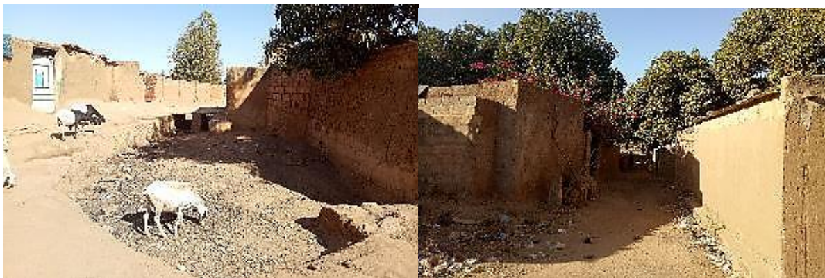
Figure 18. Sidewall protection for non-loti constructions in Toukin (left) and Kossodo (right)
