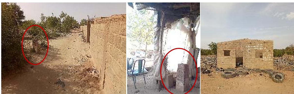
Figure 19. Boundary marker (left and centre) and suspended construction (right) in the non-loti zone of Kossodo
