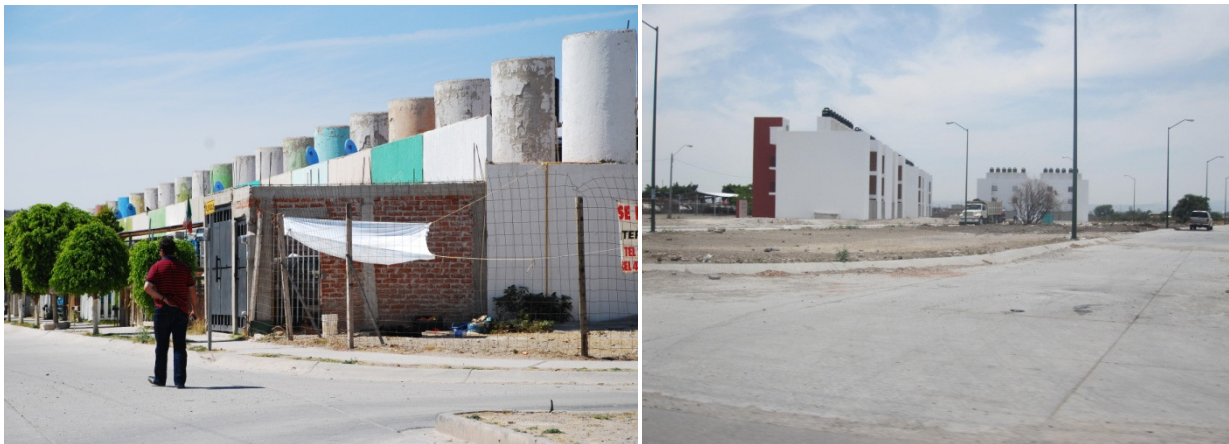
The mass production of housing is organised around low-cost models which fail to take into account the human dimension and the social conditions of the inhabitants. These great residential complexes are isolated and not integrated into a wider urban system.
