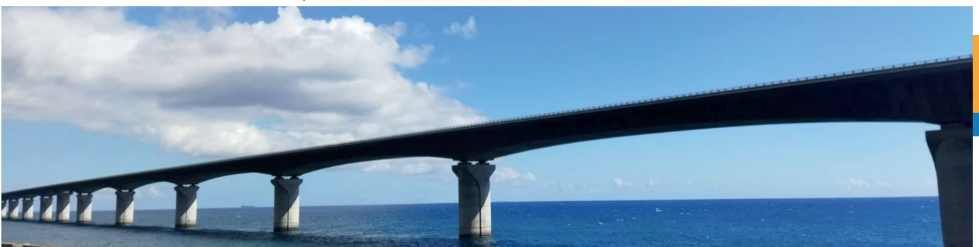
The New Coastal Road under construction, May 2021
