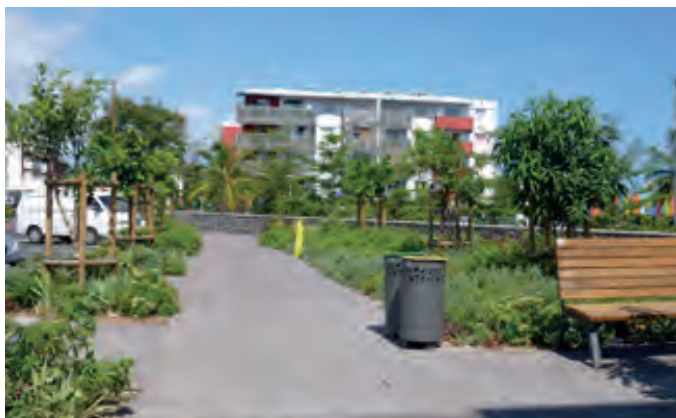
Ravine Blanche : density 50houses/ha, Sainte-Pierre Public spaces requalified with an urban park of 2ha, Source : Aymeric Delmas, Doctorant CIFRE IMAGEEN / Laboratoires PIMENT et CRENAU
