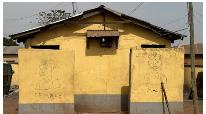
Public restrooms in Nyohini
