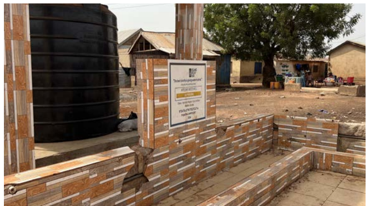
Artesian Water Well built by Islamic Relief USA
