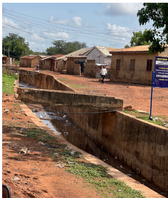
Drainage systems in Tamale
