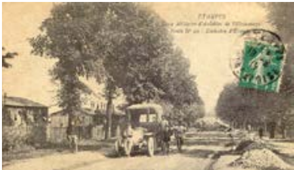
The RN20 seen from Etampes in the 1920s (Source: http://www.corpusetampoais.com/ )
