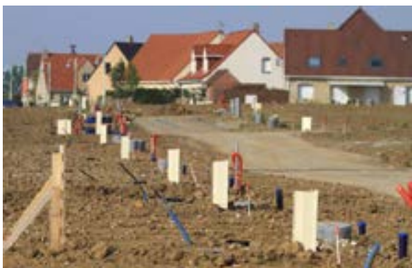
A subdivision under construction (Source: https://actualite.seloger-construire.com/ )
