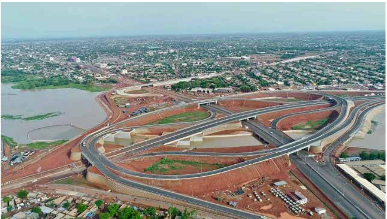
Fig 3 : The new urban road interchange
