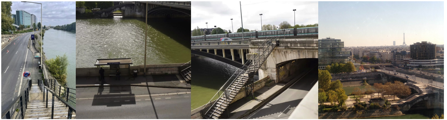
Neully bridge / RD7
