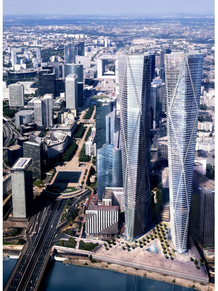
Hermitage project abandoned
