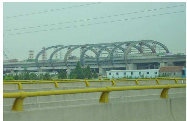
Future high speed rail station under construction
