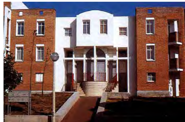
1980s-1990s: Cergy St Christophe, town buildings Source: Vincent Girard, «C'était la Ville Nouvelle», SOMOGY 2002
