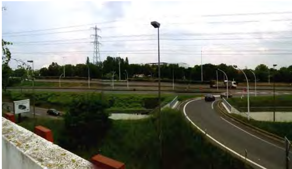
View from the A15 motorway, looking towards the Bossut barracks, from the Les Trois Fontaines car park. The tangle of roads and the division the motorway makes between neighbouring districts can be clearly seen
