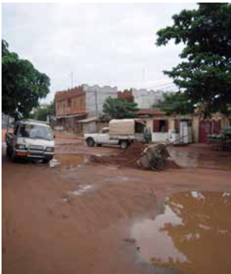
Flooded Road : Koutongbé (May 2010)
