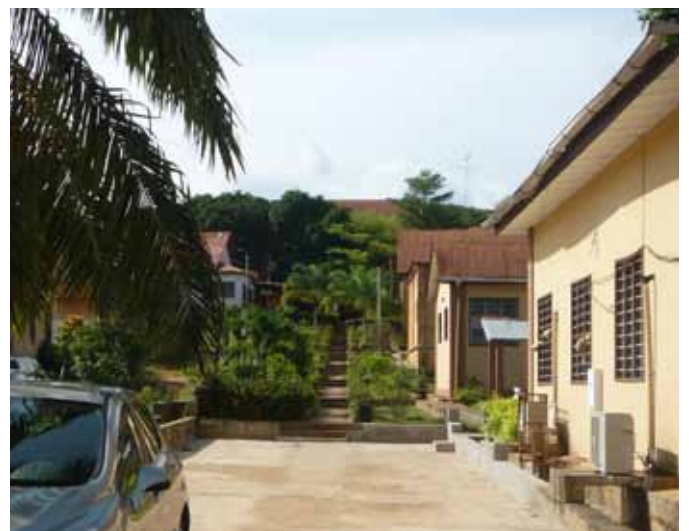
Slope incorporated in the private domain functioning as a special landscape feature, while maintaining the drainage function
