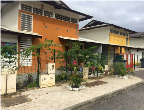
Social housing projects, « Les Hauts de Balaté » in the Saint-Louis district, in Saint-Laurent
