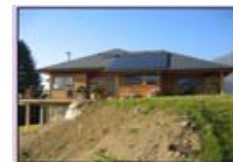
Single Family House equipped with Geosol
