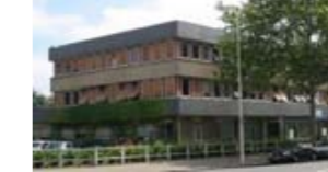
Office building in Lyon (F) before renovation
