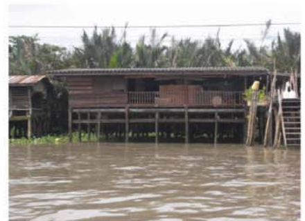
Traditional House on Stilts
