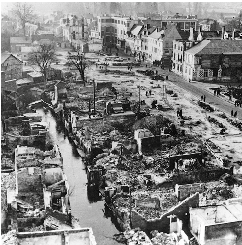
5. Evreux (27) after the German bombardments of 9-10 June 1940. One can distinguish the plots of land previously divided into individual housing units lining the River Iton.
