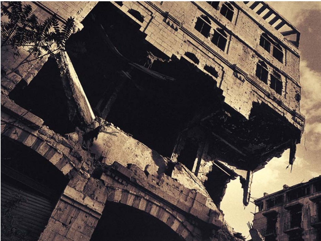
14. Beirut. Building in the city centre hit by a shell.
