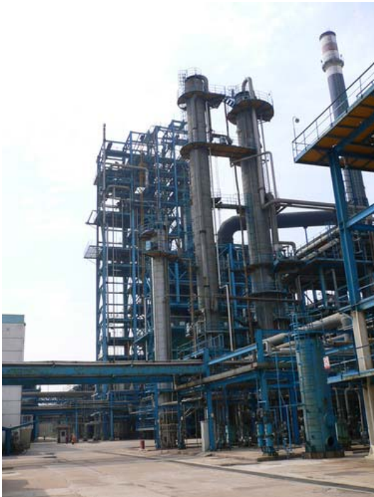
Oil distillation tower
