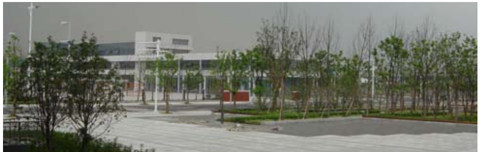
A and B Zones North Square and offices. Finished part of the project in front of the station.
