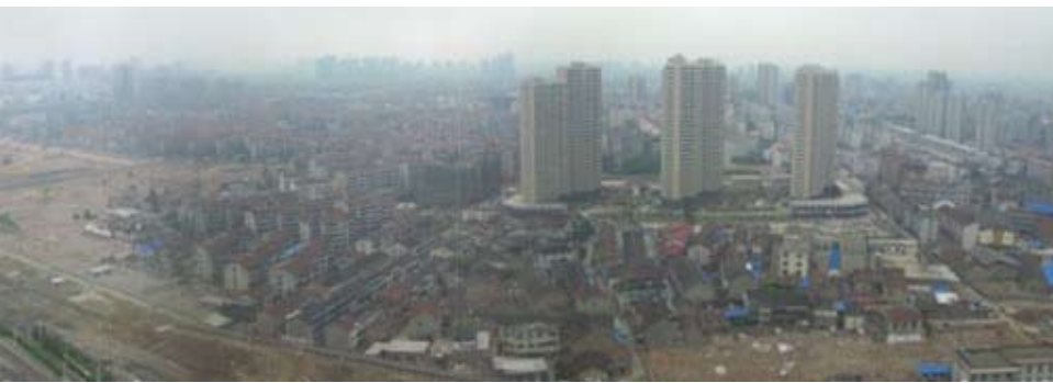
A view of the north-west part of the Central station area, before the planning of the north part.
