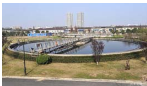
Water treatment station
