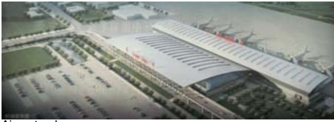
Airport enlarge project.
