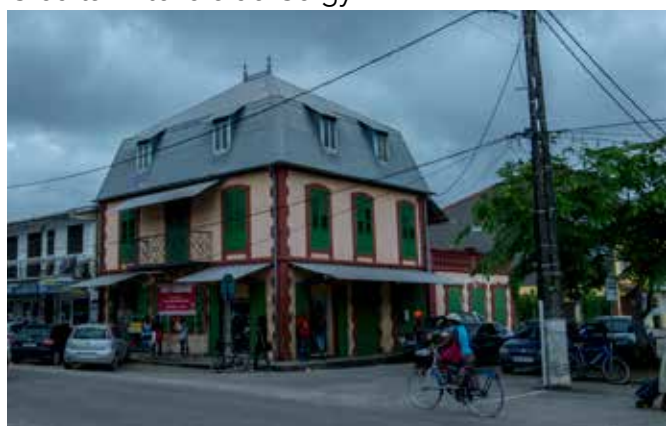
Colonial house. Credits : Ateliers de Cergy
