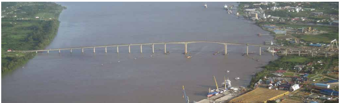
Paramaribo bridge crossing Surinam river.
