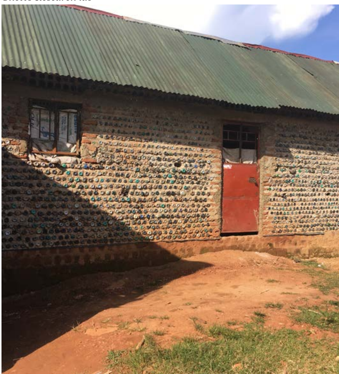
A building made with plastic bottles and plastic bags in Kamwokya by the Ghetto Research lab
