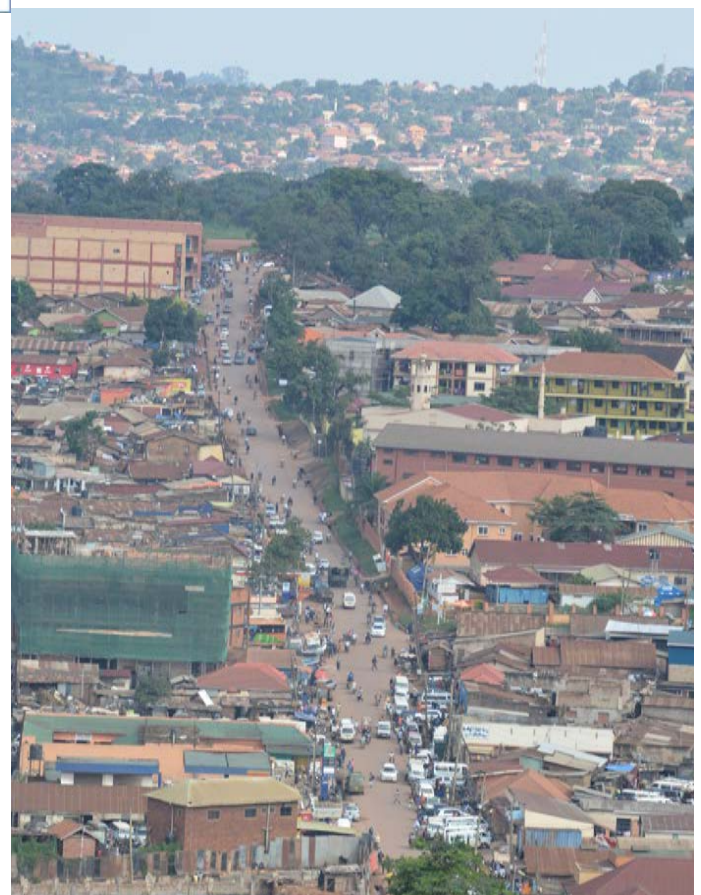
An aerial view of a suburb in Kampala with a mix of high-rise, high density buildings. (JG)
