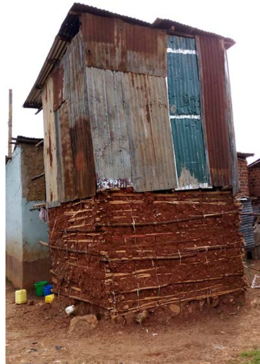
An elevated house in Namuwongo to face floods
