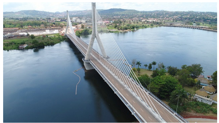
Jinja's Source of the Nile Bridge, commissioned in 2018, is an important point of the Jinja-Kampala expressway (The Independent)
