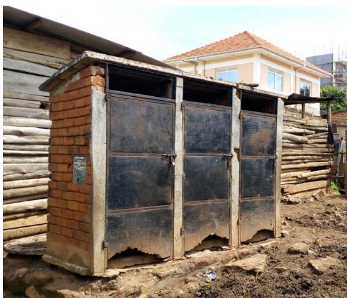
Sanitation facilities built with Interlocking Stabilised Soil Blocks in Kanyogoga
