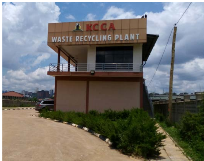
The Wankoko Waste Recycling Plant
