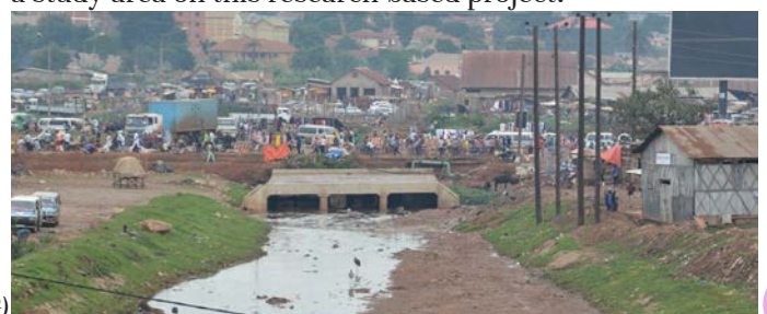
Lubigi drainage channel (JG)
