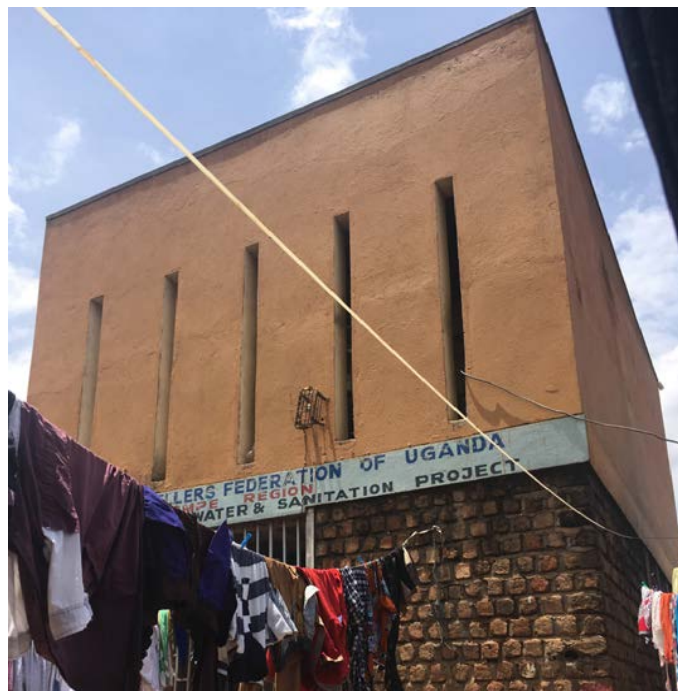
A building with sanitation facilities and public meetings room in Bwaise provided by the Slum Dwellers Federation of Uganda
