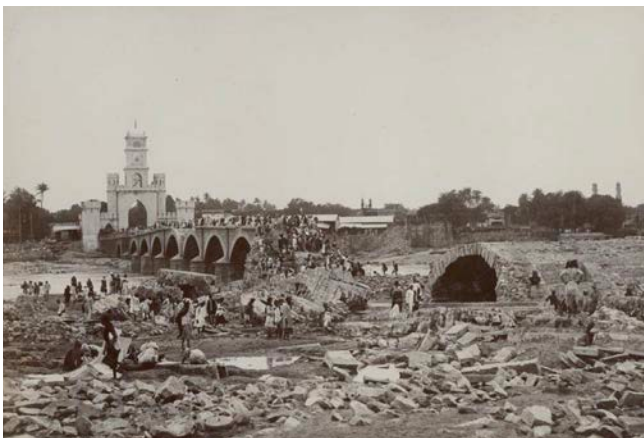
Fig 8: The Afzal Gunj Darwaza stands behind the desolated remains of the Afzal Gunj Naya Pul after the floods, 1908.
