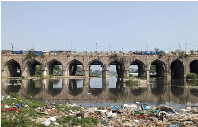
Fig 21: Musi and Puranapul bridge (source: Nithya Khendry)
