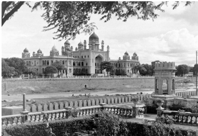
Fig 10: High Court on the southern bank of the Musi river; Kiosk on the northern bank in the foreground
