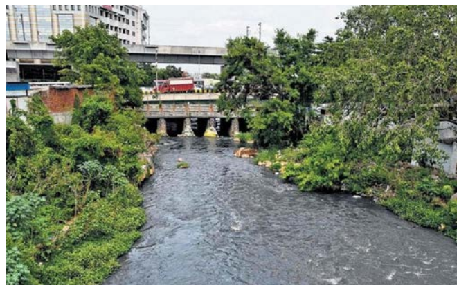
Fig 32: Open stormwater drain between the Fathenagar STP and Rain Garden in Begumpet (source: The New Indian Express)
