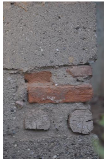
Using wood, brick and concrete together
