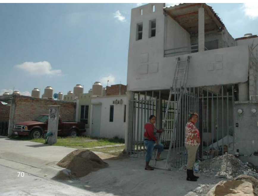
Self-made building in a social housing neighbourhood.
