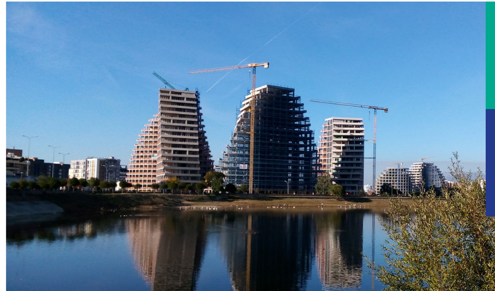
The «Lake View» residences in construction, along the artificial lake
