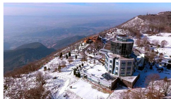
Cable-car complex (Dajti Express)
