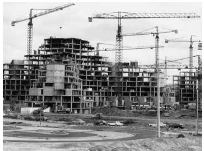
Figure 14. The new town of Évry, construction of the pyramid neighbourhood
