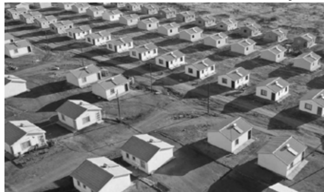
Figure 43. The single storey, stand-alone typology is the ubiquitous model for the RDP home. This model does not respond to the multidimensional needs of urban inhabitants and creates unsustainable densities (source: Vharanani Properties).
