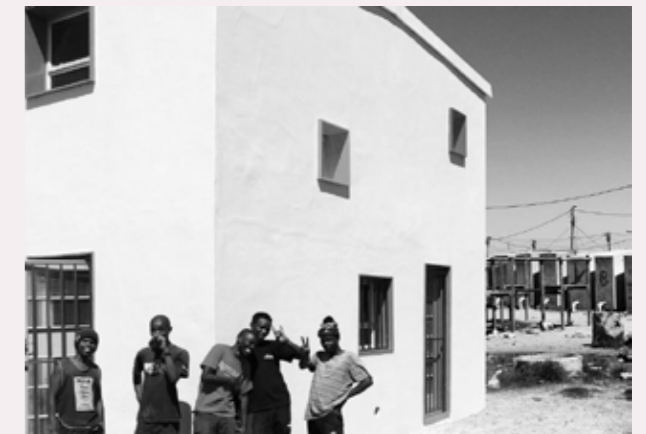
Figure 50. Two single storey semi-detached shacks were incrementally developed by UBU and Sweet Home community members to become the final product pictured here (source: UBU).
