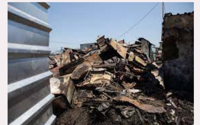
Figure 56. The devastation of a fire in Kosovo. The density of shacks, the storage of building materials between shacks, and the storage of paraffin used for cooking allows fires to spread fast through informal settlements. Fire trucks are unable to access the settlements. Ikhayalami's community-driven reblocking processes address this (source: Ground Up, 2018).
