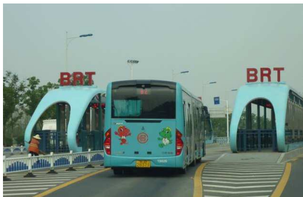
Station de bus - BRT
