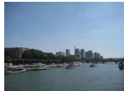
Fronts of Paris buildings along the Seine
