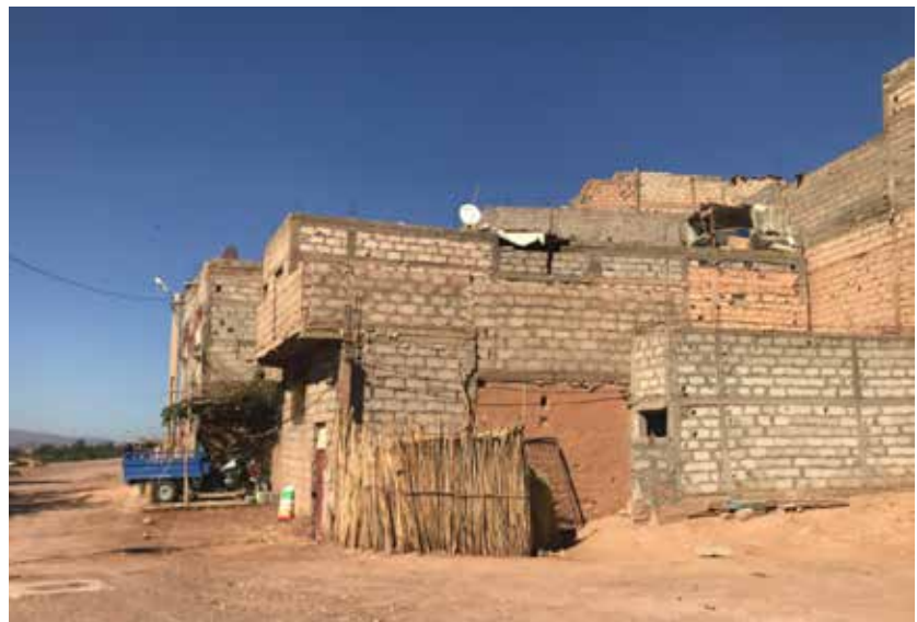
Informal housing in Ait Kdif close to the flood zone - October 2018
