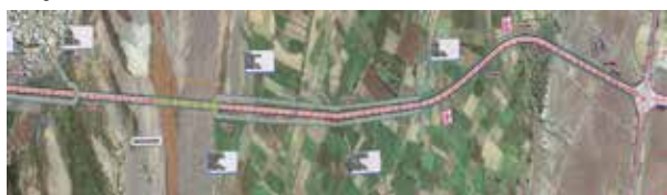
Bridge location - Al Omrane
