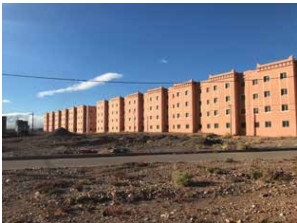
The Sidi Othmane urban centre in Tarmigt – September 2018
