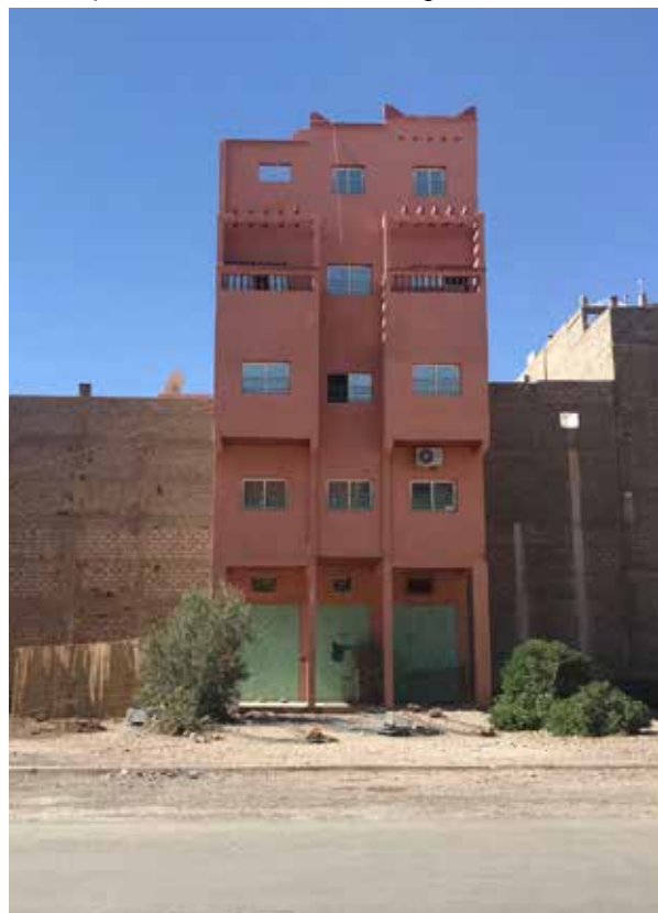
Typical building in a neighborhood under construction near Al Whada - October 2018
