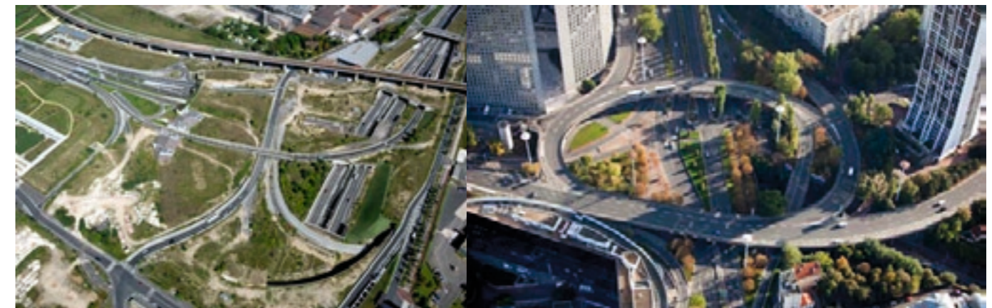
The territory's transport infrastructures, the scales superimposition. Source: Flickr CG92 et DREIF
