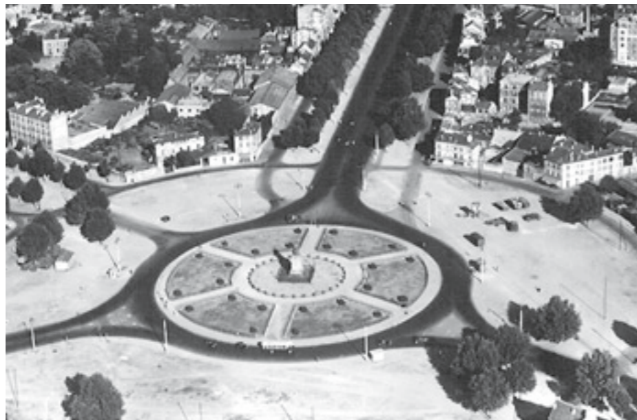
The launching of the operation
