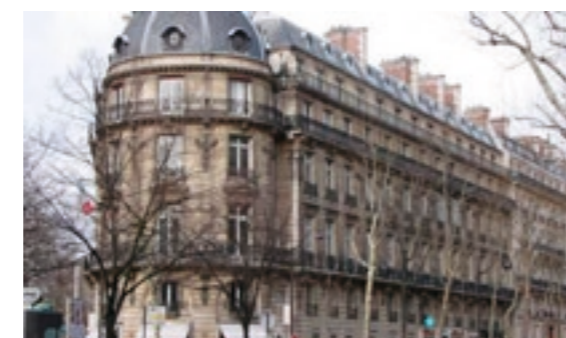
Example of Haussmann building in the QCA Source: http://www.constructa.fr
