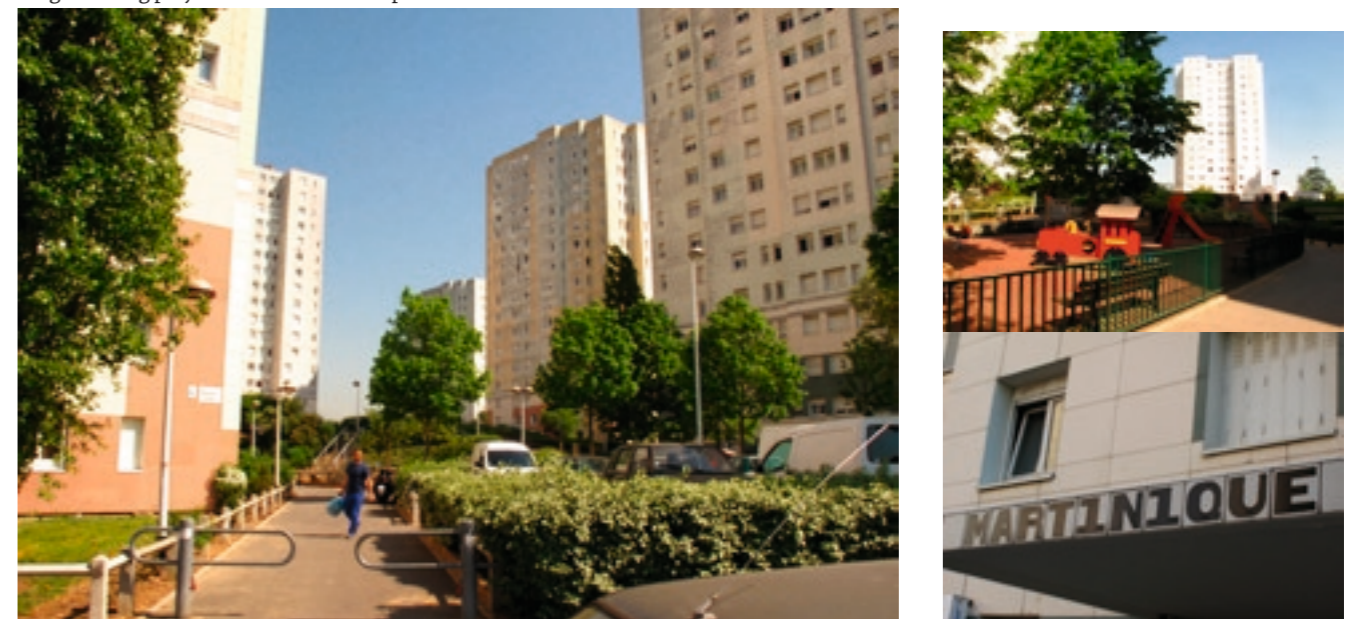
Large housing project from the inside: pedestrian paths, green areas, playgrounds.
