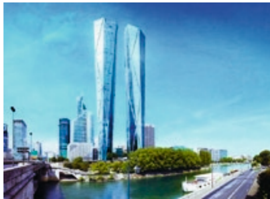
The Hermitage towers. Source: http://www.ladefense-seine-arche.fr
