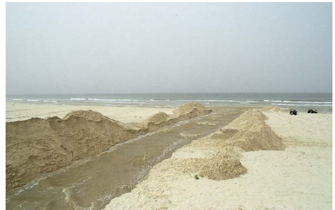
Opening the load-shedding channel; Source : Photo CRDS.
