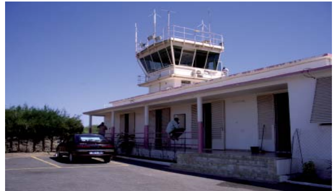
Control Tower and technical unit
