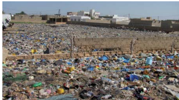
Plot surrounded by a wall and backfilled with waste.
