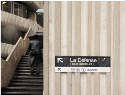
Access to the elevated plaza
